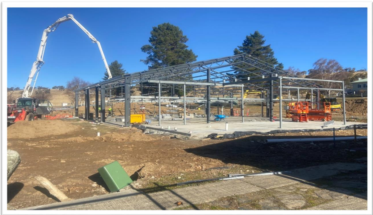
Current rebuild of hatching shed area (as of 1 st July 2023)
